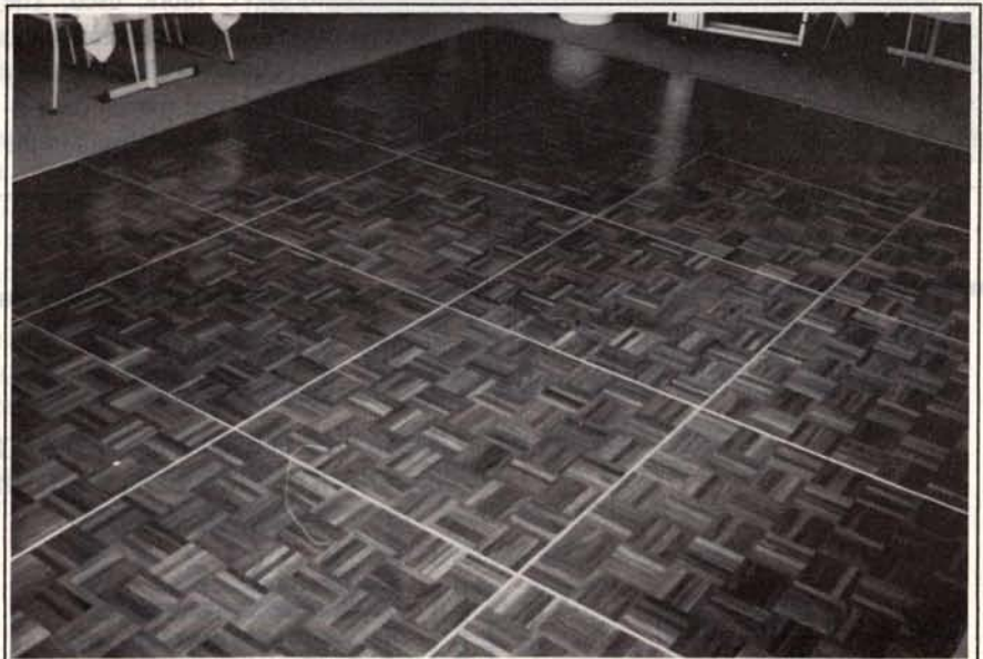
Australian Portable Dance Floor sections are made of beautiful finger parquet, finished to a very high standard and fixed to a medium density moisture resistant craftwood.
